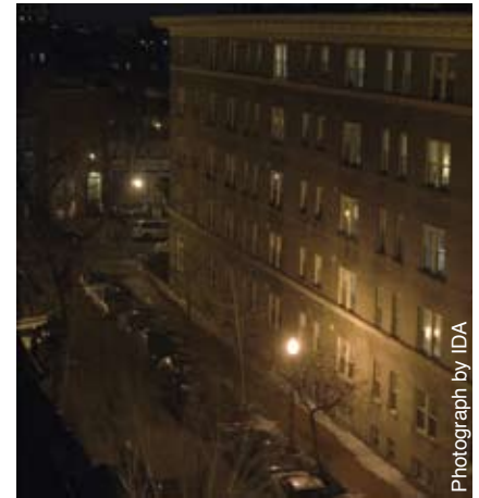
Light trespass, Washington, DC. This "street lighting" directs very little light onto the street. Instead, it sends wasted light into the sky and the sides of residential buildings where it may not be needed or wanted.
